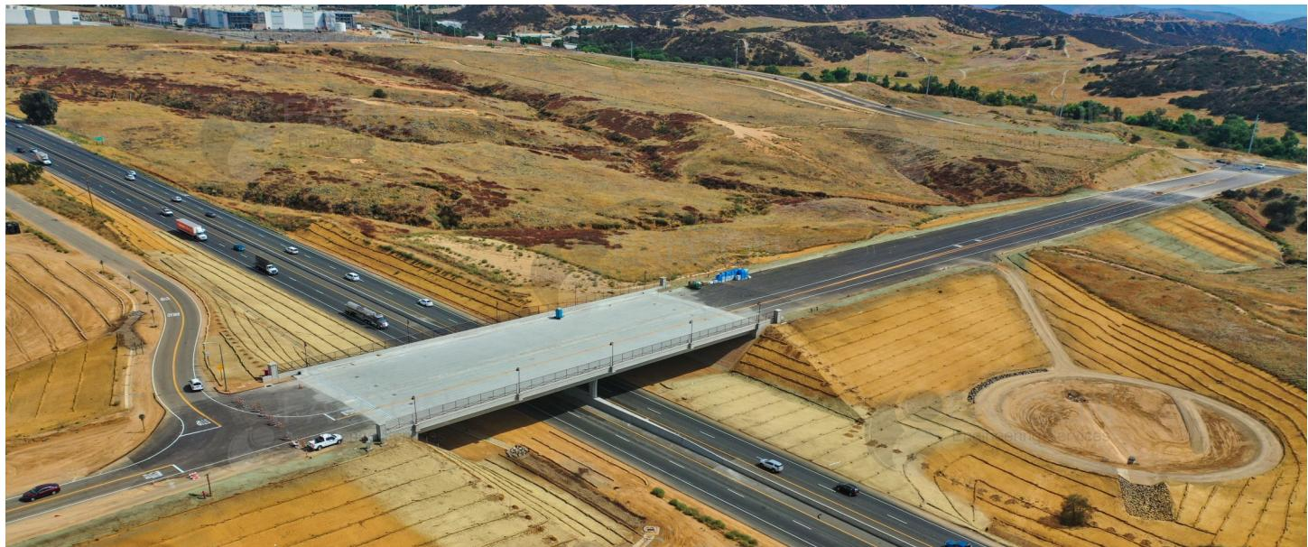
The phase 1 of the Potrero Interchange is nearing completion over SR60. Once open, the overcrossing will provide access from Oak Valley Parkway to 1st Street. Design Plans for Phase 2 of the project, which include on and off ramps, are 95% complete. Funding for the ramp phase includes a pending application for a BUILD grant through the Department of Transportation (DOT). Notification of award is expected by mid-November.
