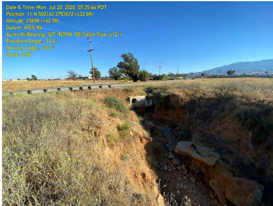
PHOTOGRAPH 1: The upstream portion of Feature A where the culvert begins the feature beneath Pennsylvania Avenue.
