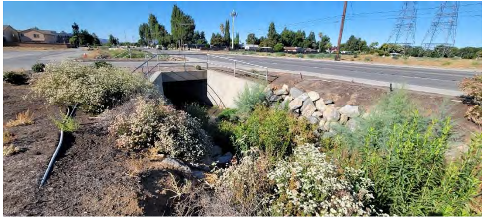
Photograph 9: Looking southwest with a view of a driveway leading to a parking lot within the electrical easement, passing over a culvert with riprap.
